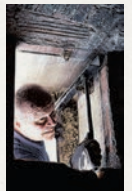
Engineer and facilities director Yordan Kovatchki climbs to the top of the historic dome at OLV.
